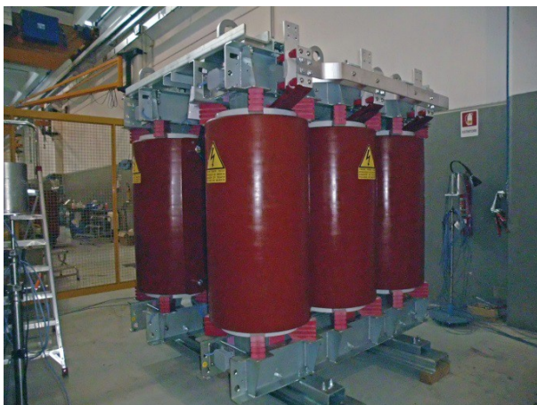
SEA Laboratories, the FPPCC PS transformer tested
