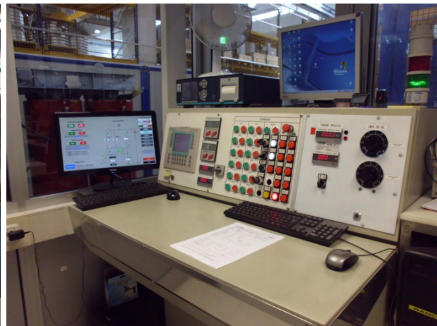
SEA Laboratories, the test hall
